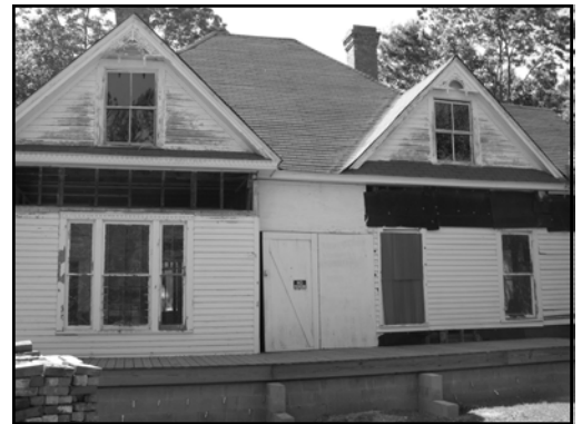
Duncan/Strickland Home prior to renovation Photograph courtesy Margaret Lynne Ausfeld
