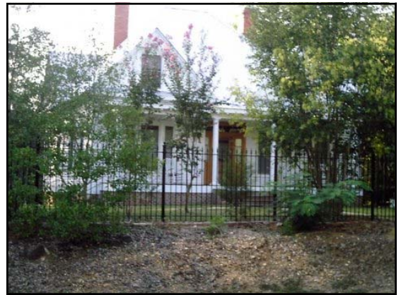
Duncan/Strickland Home after to renovation. Photograph courtesy Gary Burton
