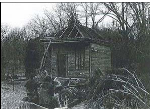
Moving day for medical office. Photograph courtesy Old Alabama Town
