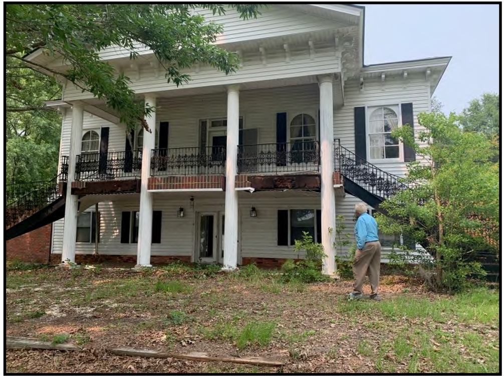
The Suggs' House in its current, vacant state on West McLean Road, photo courtesy Tony Hopper.
